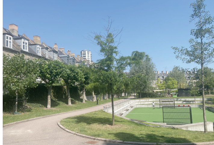
Carlsberg area in Copenhagen with new green urban spaces capable of detaining rainwater to decrease the risk of flooding and simultaneously be used for recreational activities.
