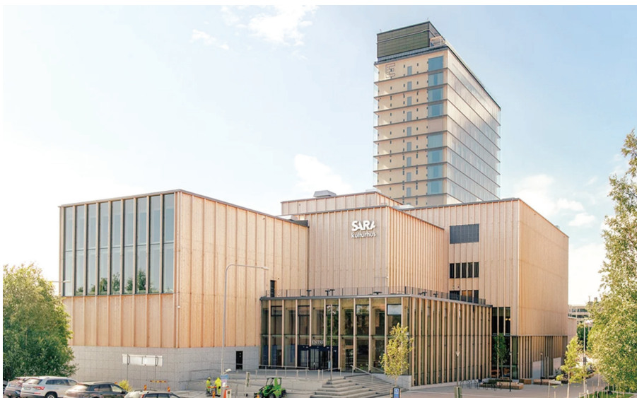
Sara Kulturhus, cultural center and hotel, constructed in wood in Skellefteå, Sweden.
