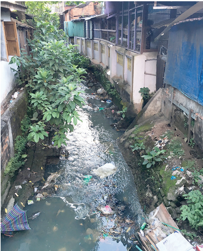
River clogged with waste while adjacent buildings are in risk of flooding.
