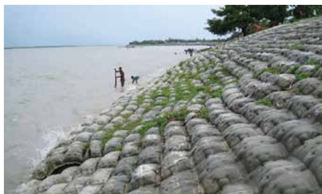
Figure 43: Example of bank erosion protection through revetment composed of sand-filled geotextile bags
