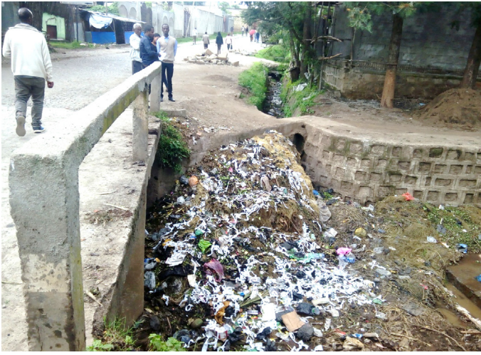
Solid waste dumped at the riverbank, causing pollution of the water (often used for drinking and cleaning), clogging drainage channels causing flooding during rainy season, odour, vermin etc.
