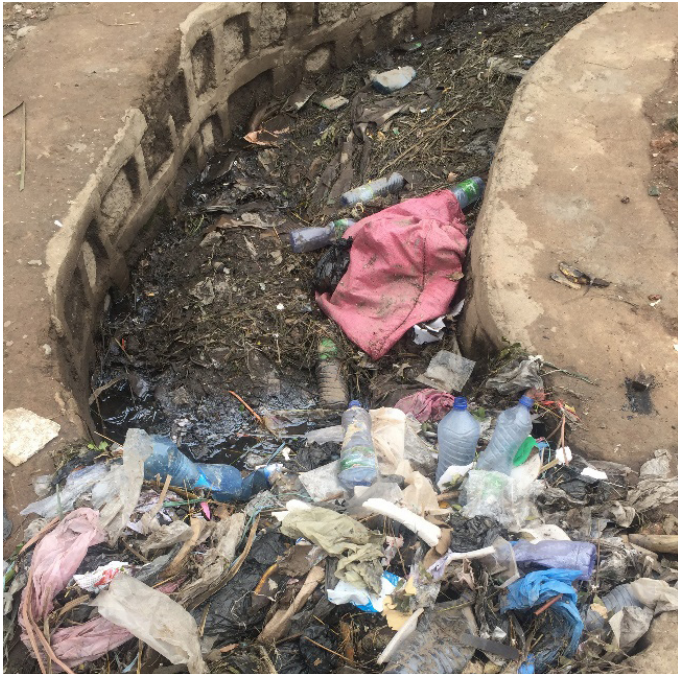
Above: Clogged drainage in central Shashemene.
