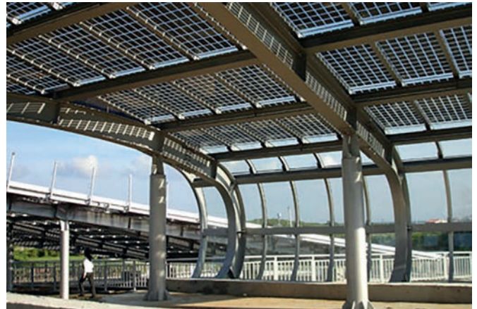
Figure 24: Solar photovoltaics roof making Kannar Market a net energy producer
