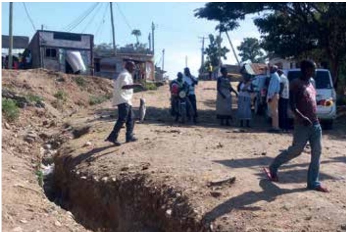
Eroded dirt road (top) and pit latrines at a school (under)
